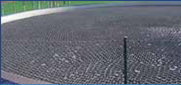
SLURRY STORE COVERS
